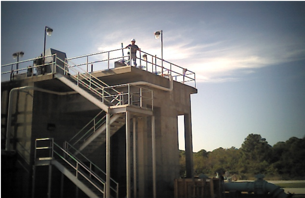
Figure 2 - Northwest Regional Water Reclamation Facility Headworks
